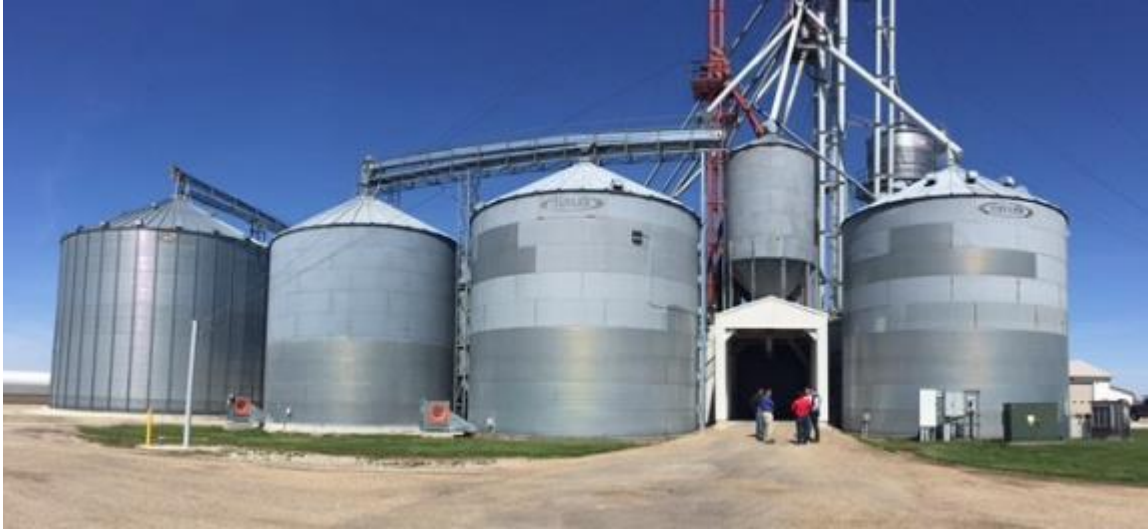
Figure 4: Gingerich Farms on-farm storage, Illinois, USA. Source: L. Allen, July 2016
